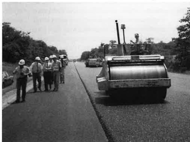
Compaction of SMA with standard steel wheel roller (non-vibratory).
