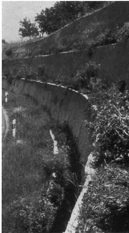
Completed, permanent soil-nailed wall along highway in Germany. Tiered to allow plantings, it is known as a "greening" wall. Wall facing is dry-mix structural shotcrete left-in-the-gun finish.
