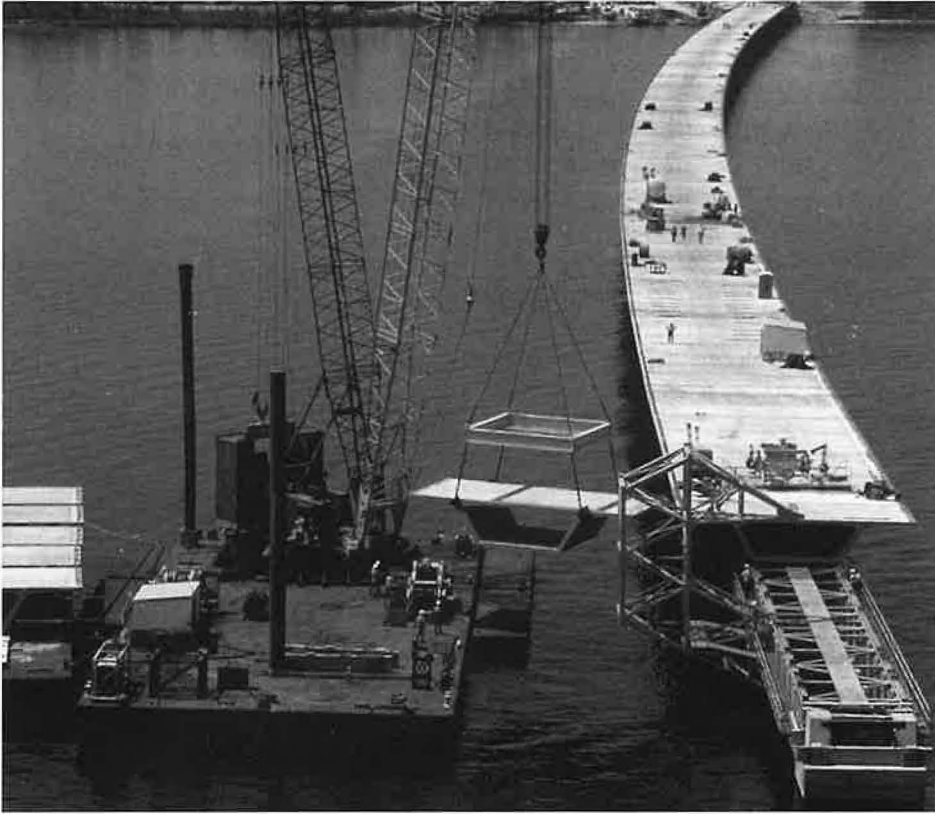
Choctawhatchee Bay Bridge links Destin and Bluewater Bay in Okaloosa County in northwest Florida panhandle. Completed five months ahead of schedule, bridge was constructed by Traylor Bros., Inc., under $42.5 million contract with Mid-Bay Bridge Authority. The 3.6-mile post-tensioned box girder bridge, designed by Figg Engineering Group, was constructed with precast segments.
