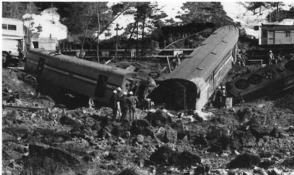
FIGURE 3 Landslide that resulted in derailment of California Zephyr passenger train near Granby, Colorado, in April 1985. Landslide began as an earth slide through the base of the railway embankment ( middle background ) and rapidly moved some 70 m (200 ft) as a debris flow, partially damming Fraser River ( foreground ).
