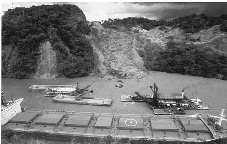
FIGURE 5 October 1986 reactivation of Cucaracha Landslide in Gaillard Cut, Panama Canal. Landslide extended nearly across the canal, but much of the toe had been removed by dredges by the time photograph was taken.
