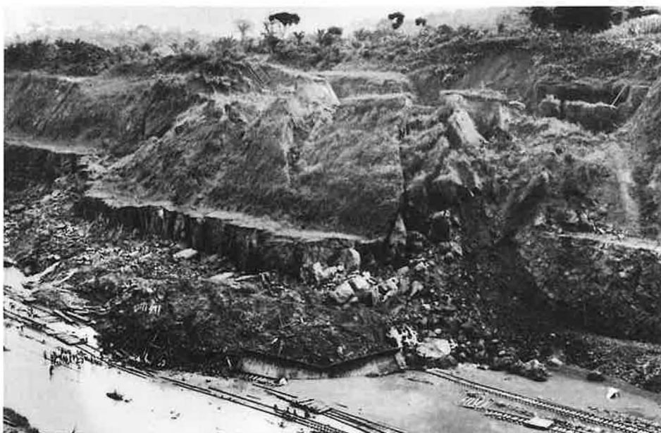
FIGURE 4 Cucaracha Landslide in Gaillard Cut, Panama Canal, August 1912. Note railroad tracks and cars destroyed by this 230,000 m 3 (300,000 yd 3 ) slump.
