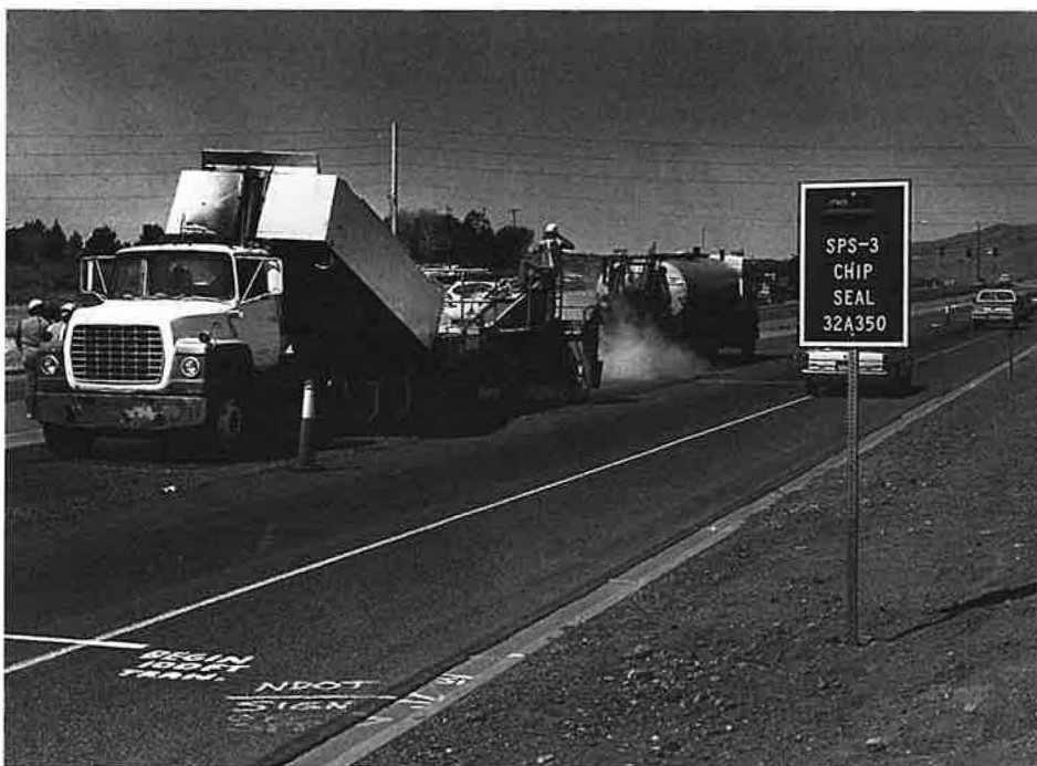
Workers lay chip seal in Sparks, Nevada, as part of SHRP study to evaluate performance of various maintenance strategies for asphalt pavements.
