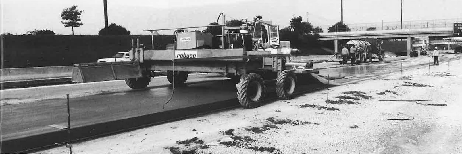
Equipment used to finish surface of experimental section.
