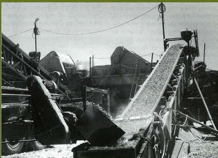
Concrete recycling operation on I-84 in Idaho.
