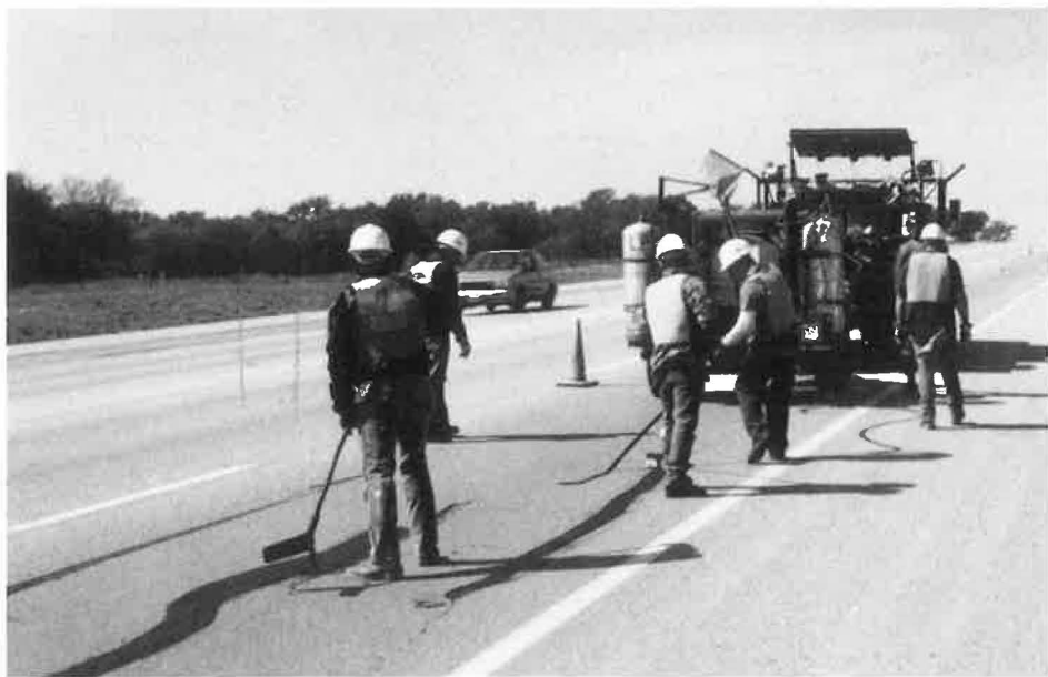
FIGURE 1 Conventional crack-sealing methods.
