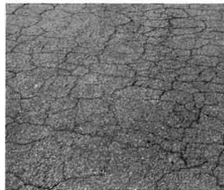
FIGURE 2 Old asphalt pavement with surface cracks but with good structural integrity is suitable for hot in-place recycling.
