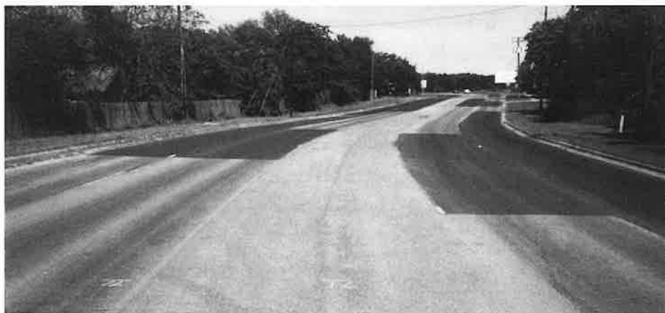
FIGURE 3 Patchwork surface is unsuitable candidate for hot in-place recycling because of difficulty of controlling mixture design.
