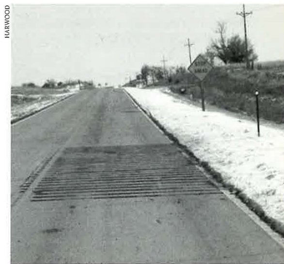
FIGURE 1 Typical raised rumble strip in roadway on intersection approach.
