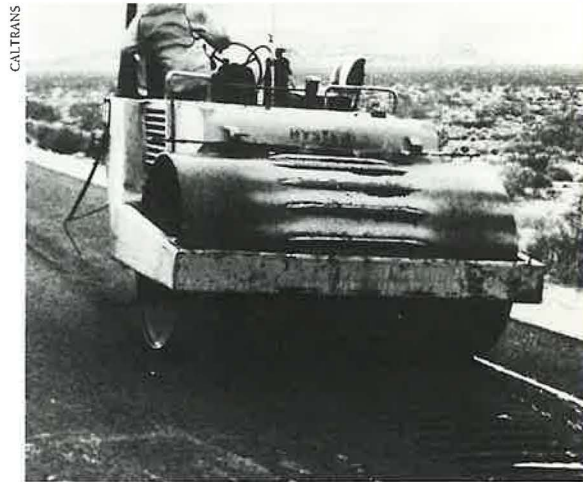
FIGURE 4 Roller being used to place rumble strips on asphalt shoulder.
