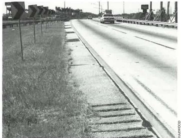
FIGURE 3 Shoulder rumble strips on narrow bridge approach.
