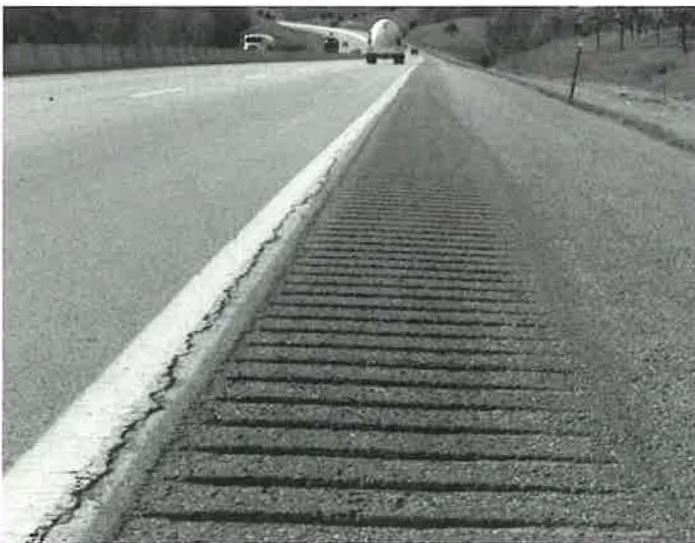
FIGURE 2 Continuous rumble strips on asphalt shoulder.
