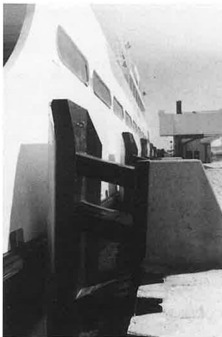
New high-technology composite marine fenders outperform traditional materials in energy absorption and are immune to marine wood borer attack.
