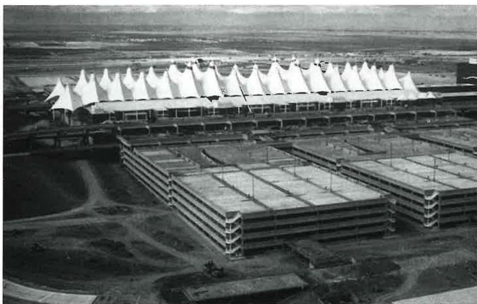
Parking structure at Denver International Airport is predominantly precast concrete containing corrosion-inhibiting admixture to help increase service life.
