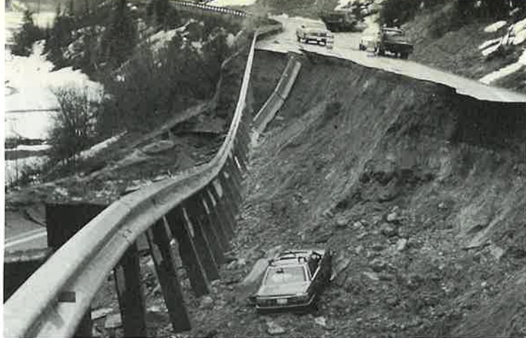
Destruction of Colorado State Highway 133 by April 1993 landslide near Paonia Reservoir, western Colorado. TAYLOR/COLORADO STATE PATROL
