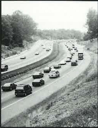
Interstate 476 in Pennsylvania is the site for Traffic and Incident Management System.
