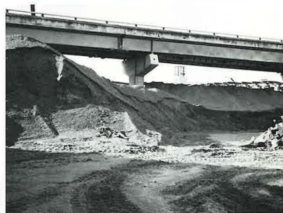
Demolition activities related to reconstruction of Cypress Freeway in San Francisco (top), after Loma Prieta Earthquake in 1989 afforded Caltrans an opportunity to recycle several types of material, including reinforcing steel bars (center) and concrete rubble (bottom).
