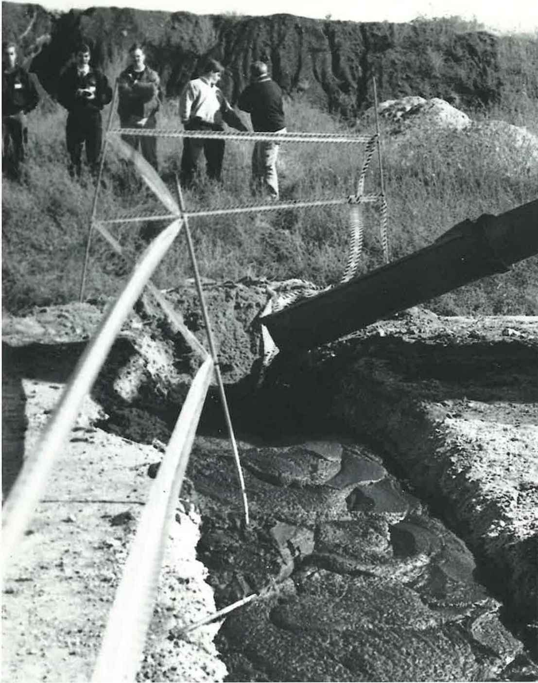
Spent green sands from ferrous castings can be used in place of natural sand in flowable-fill mix.
