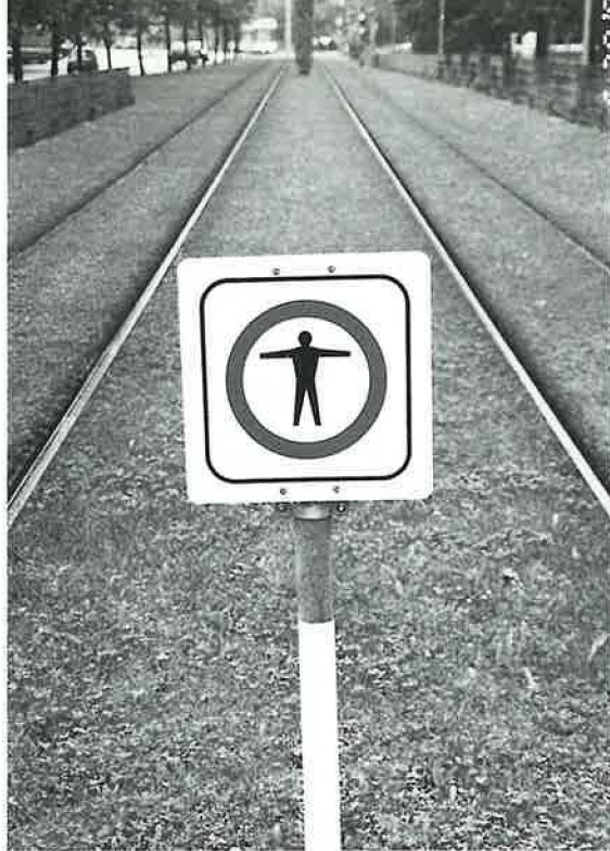
Grassy, parklike right of way for light rail in Freiburg, Germany, with pedestrian warning sign.
