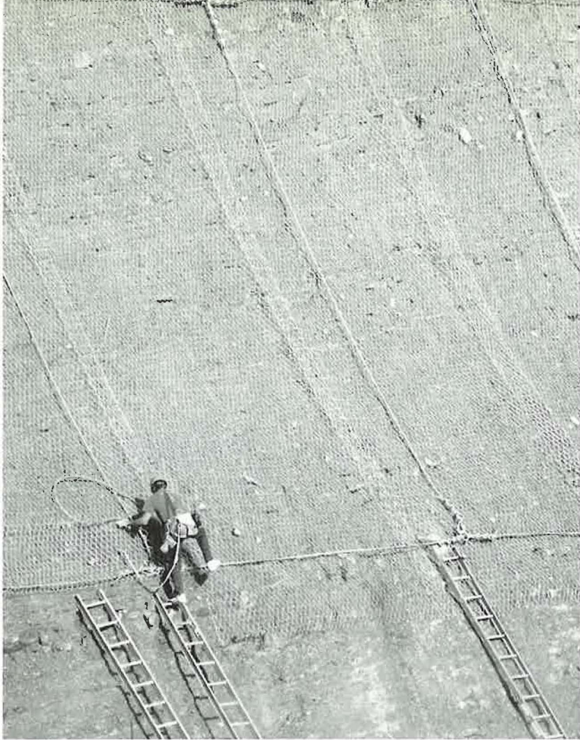
Worker installs special netting to prevent rocks from falling into roadway along I-75, Kentucky.
