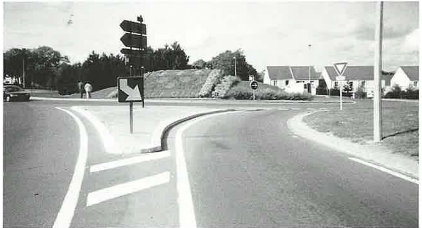
Top: Pavement marking of roundabout in Washington, D.C., is not well defined.
