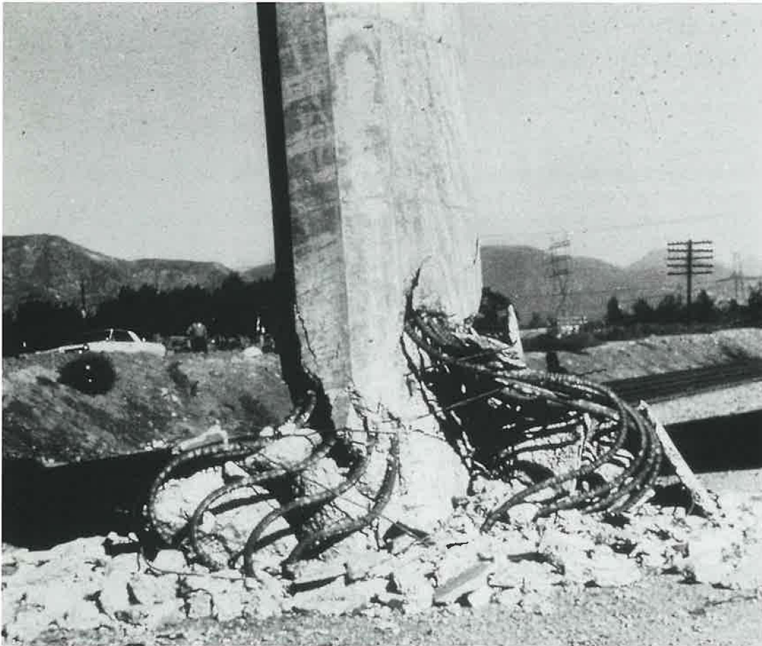
Plastic hinge confinement failures ( above ) and column shear failures ( right ) were among the damage suffered by bridges in the 1971 earthquake in San Fernando, California.
