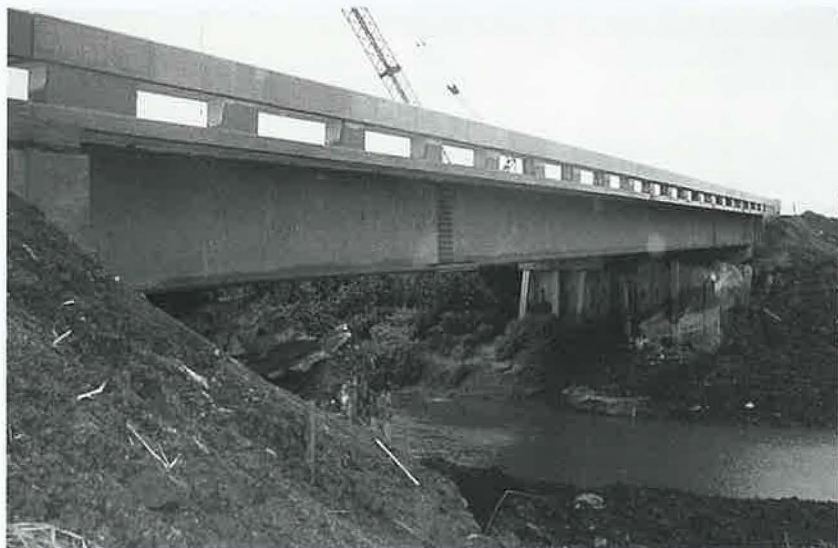
The Snyder South Bridge in Nebraska is the first U.S. bridge constructed from high-performance steel.
