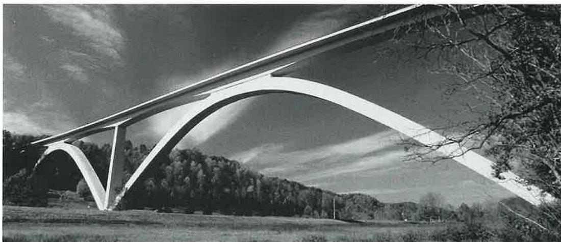
Completed Natchez Trace Parkway Arches, designed by Figg Engineering Group, with 582-foot arch span, and measuring 155 feet from Tennessee Route 96 to top of bridge. Predominant span is 246 feet variable depth. Piers are tapered, and arch varies in depth.
