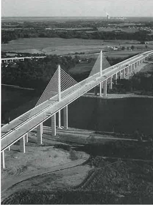
The Chesapeake & Delaware Canal Bridge, a precast segmental superstructure with a 750-foot cable-stayed main span, is located in St. Georges, Delaware.
