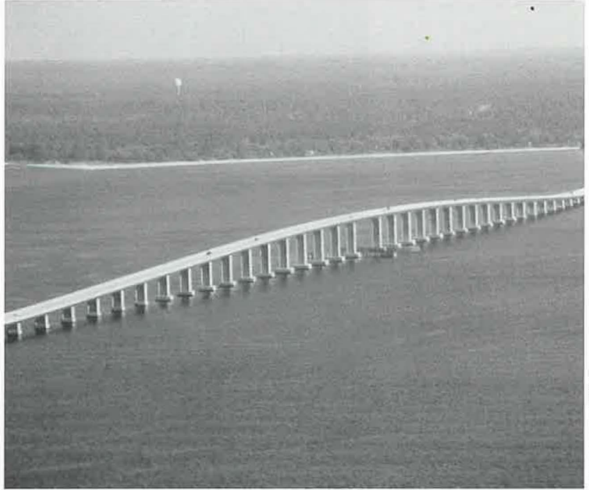
The Mid-Bay Bridge, a precast segmental superstructure with a 225-foot main span, is located on Choctawhatchee Bay in Okaloosa County, Florida.
