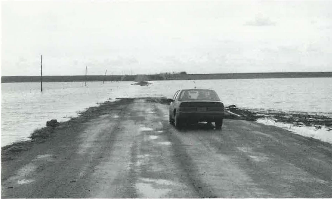
Flood conditions in South Dakota, April 1997. The unusually wet spring and winter months of 1996–1997 resulted in major problems for transportation agencies in several regions of the country.
