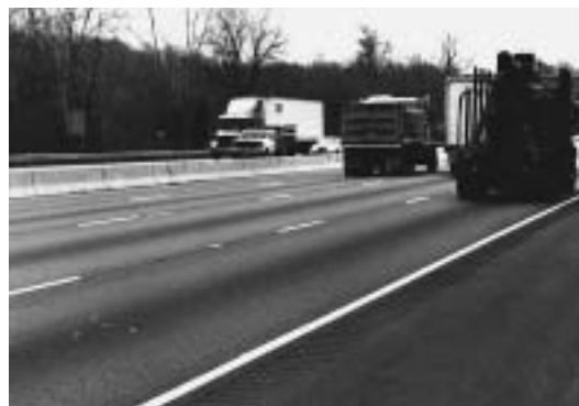
After 7 years of service with the top 4 inches of surface replaced, New Jersey I-287 remains in good condition today.
