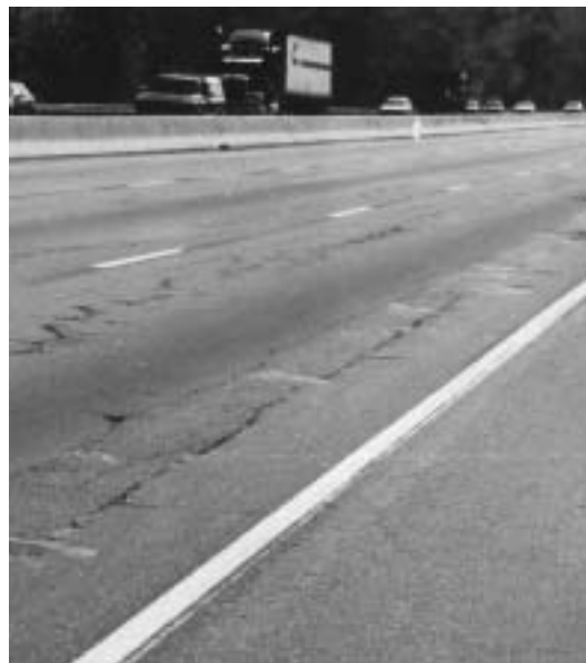
In 1993, after 26 years of service, New Jersey I-287 (above) appeared to be in terminal condition.
