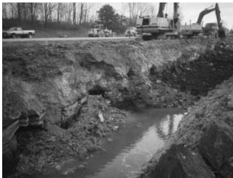
Eighteen-foot trench after excavation of the overburden and mined coal seam. Note the exposed mine openings.
