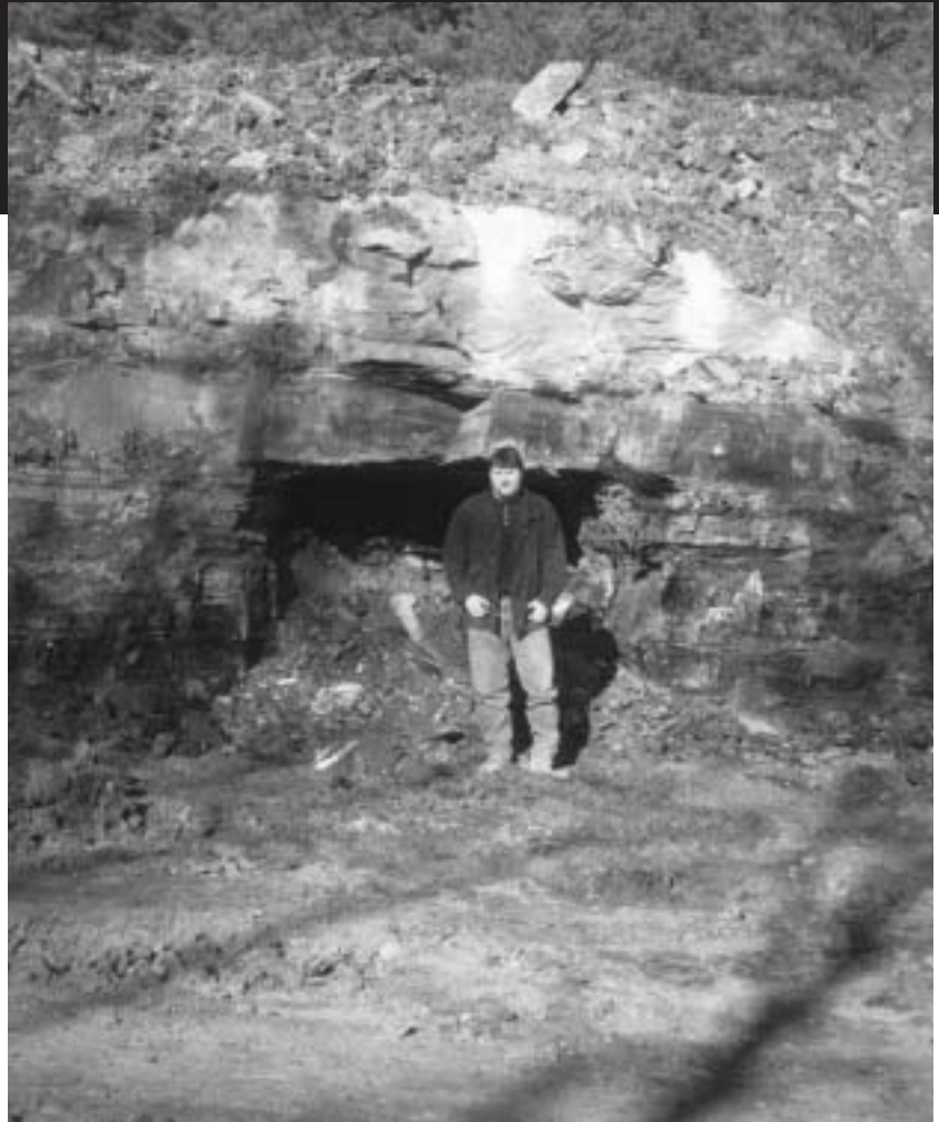
Ohio DOT employee in front of four-foot-high void discovered underneath eastbound lanes of State Route 32.
