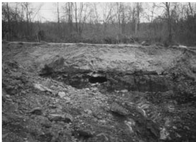
Exposed mine void beneath State Route 32.
