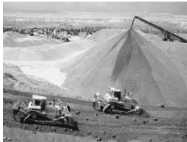
Alternate aggregate source material, suggested by value engineering program, played important role in construction on NM 44.
