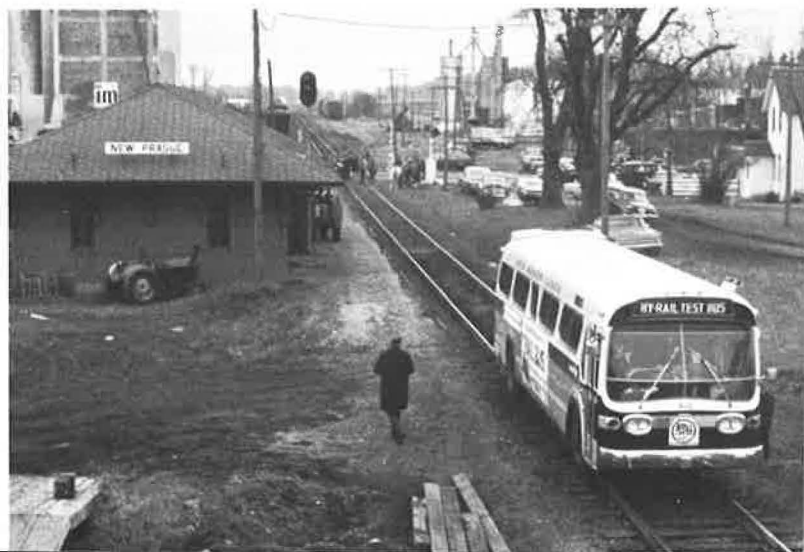
Hy-Rail test bus leaves the station at New Prague, Minnesota, on the Chicago and North Western railroad in 1967.
