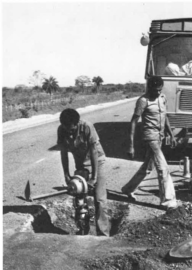
1 Cores of asphalt taken from Brazilian highways will be tested in the central project laboratory.
