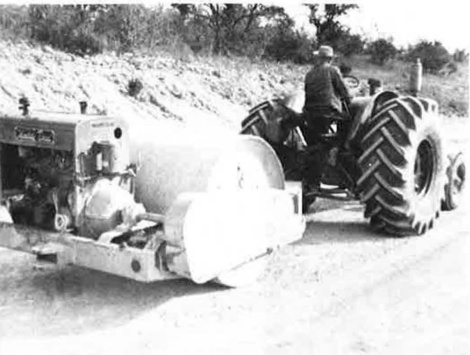
1 A vibratory roller compacts a lime-treated base at Fort Hood, Texas. This road was built 20 years ago and is still giving good service.
