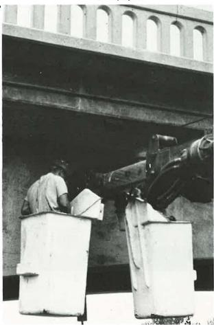
that contributed to the original crack, i.e., insufficient stirrup reinforcing steel. When the bridge is subjected to truck traffic and environmental loads, there is a significant relative motion between the two interfaces of the crack; structural rebonding is therefore difficult. If there is crack motion, the sealant epoxy is prone to crack and leak during injection; in addition, this motion may have an effect on epoxy while it is in the process of polymerizing.
