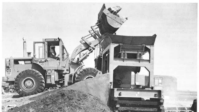
grade. Then a 6-in filter course of the recycled coarse aggregate was placed and compacted. On the filter course, a 6-in layer of econocrete base was placed by a slipform paver. Since the coarse aggregate for the new concrete had to be hauled from Miami, the economic gain from recycling the old pavement is obvious.
