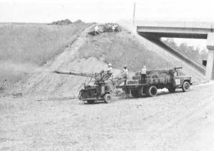
3 Protection by a diversion ditch is reinforced by mulching and seeding the slope.
