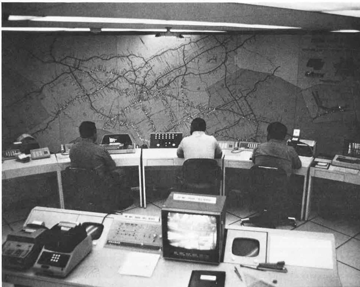
Caltrans' Operation Center in Los Angeles features a map of the area's 700 miles of freeways. Green, yellow, and red lights indicate status of traffic flow on each segment.
