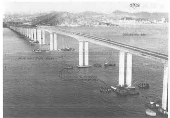
Figure 5. Prestressed box girder approach spans.
