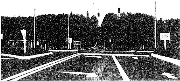
Figure 12. Poor visibility of lanes across median at wrong-way entry site.
