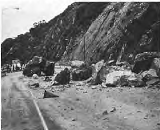
Figure 2. Rock slide on Pacific Coast Highway, April 13, 1980.
