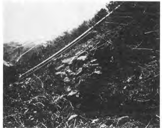
Figure 7. Surface extensometer installation.
