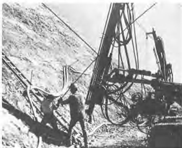
Figure 13. Dowel placement.
