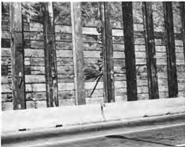
Figure 10. H-pile catchment wall and fence on Pacific Coast Highway.
