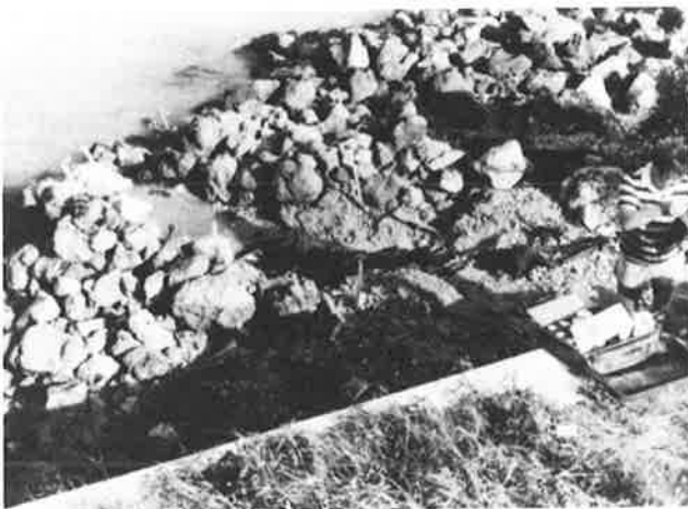
Figure 4. Excavated section at bridge abutment corner at site 1.
