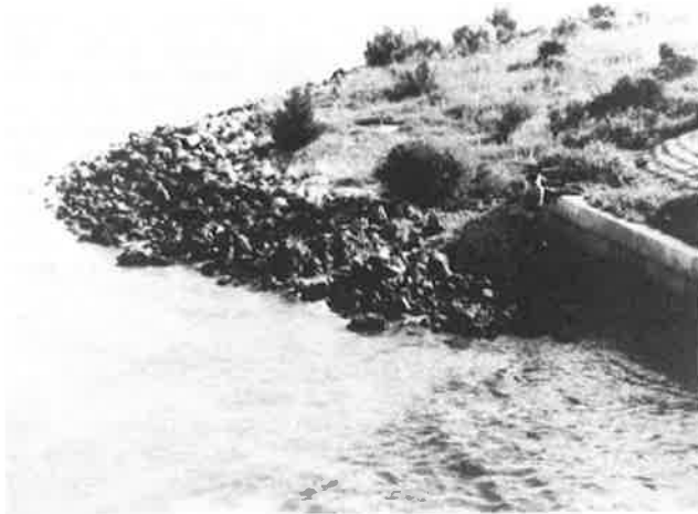
Figure 3. Limestone rip-rap covering fabric at site 1.
