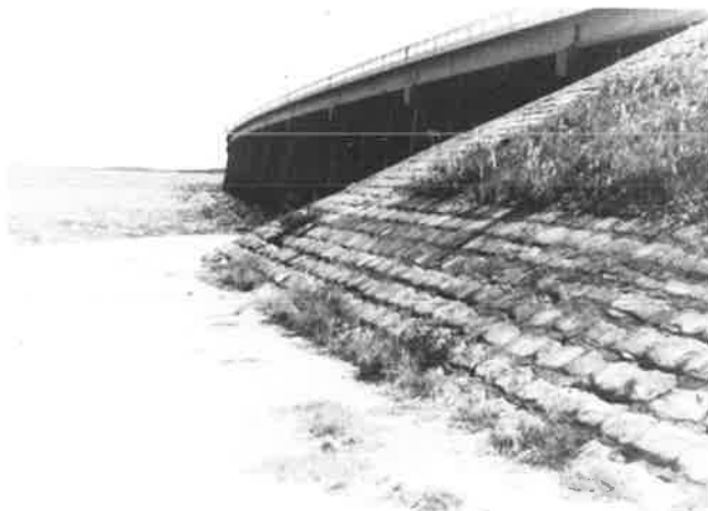
Figure 13. Armoring system: bridge side slopes and top of seawall, Bahia Honda Bridge.
