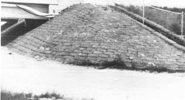
Figure 13. Armoring system: bridge side slopes and top of seawall, Bahia Honda Bridge.
