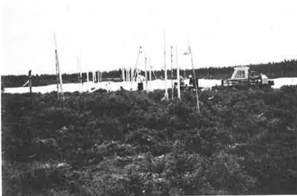
The test fills at NBR-2 were built to a height of 1 m above the muskeg surface. The final thicknesses varied from 2 to 3 m. The following is a description of the NBR-2 test fills.
