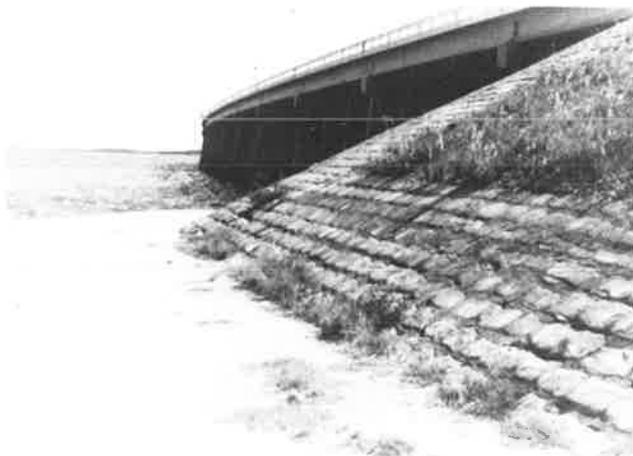
stability of the sand-cement constructed facilities, as shown in Figures 12 and 13. No erosion problems were apparent at any of the drains, slopes, and seawalls protected by the sand-cement armoring system, which indicated that the installation was functioning as designed. The armoring, in most cases, has held up completely. Some surface wear was noticeable; however, no washouts of the rip-rap were observed.
