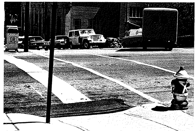
Figure 4. Curb ramp problem: ramp located out of crosswalk.
