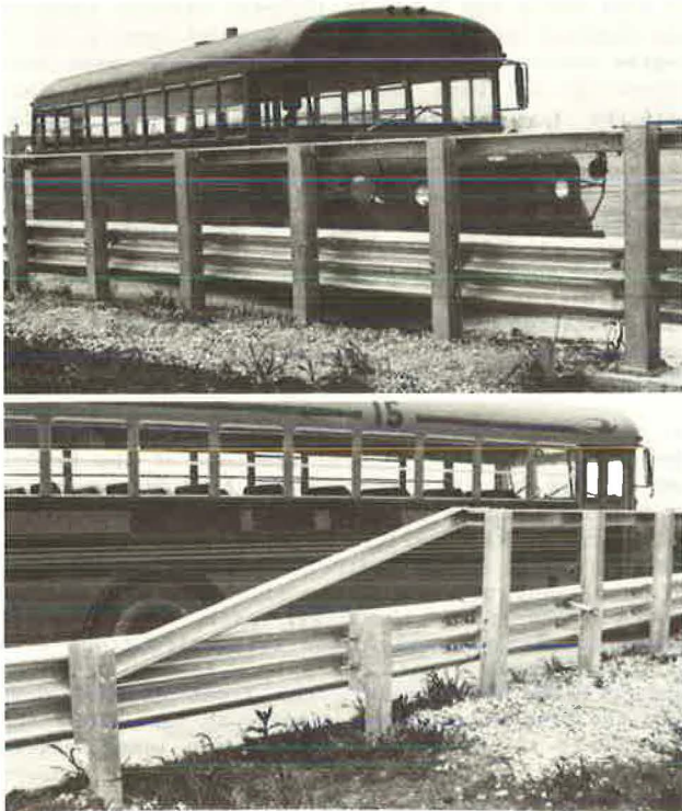
Figure 8. High-performance retrofit approach guardrail.
