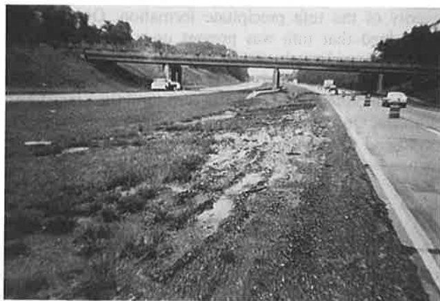
FIGURE 5 Tufa precipitate at edge of shoulder.
