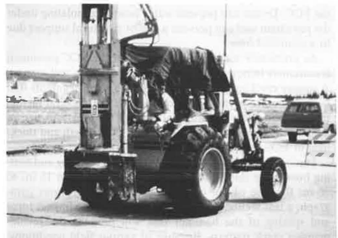
FIGURE 4 Hydraulic impact hammer for cracking PCC slabs.
