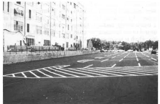
FIGURE 3 Completed asphalt concrete pavement.
