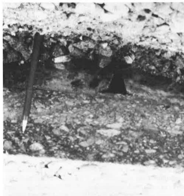
FIGURE 8 Cut-away section of asphalt overlay over a PCC pavement joint (ballpoint pen shows scale).
