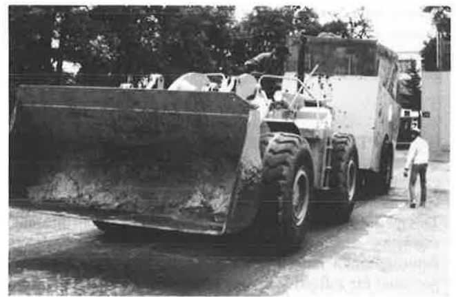
FIGURE 2 Fifty-ton pneumatic-tired roller used to seat cracked PCC pavement.
