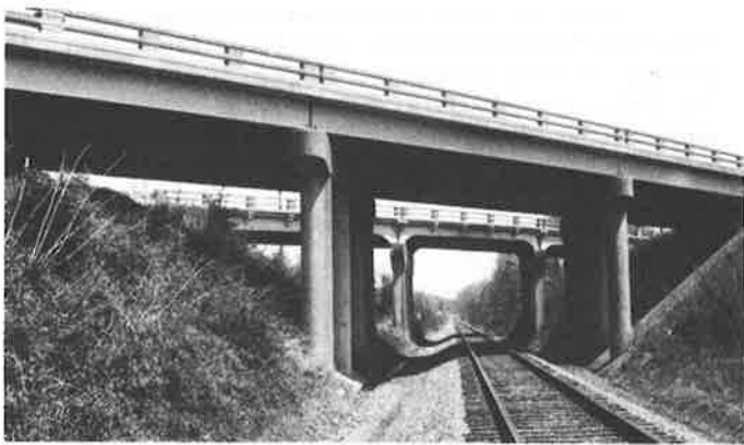
FIGURE 2 Photograph of 3 span skewed concrete bridge
