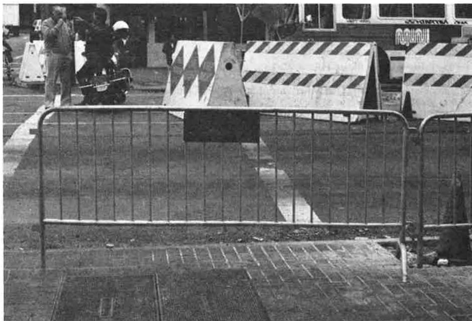
FIGURE 3 Pedestrian channelizing rails used in San Francisco.
