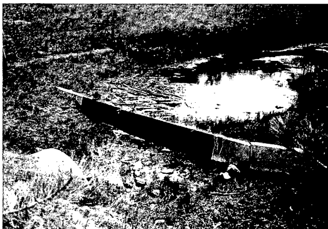
FIGURE 4 Jersey barrier plug installation.
