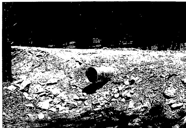
FIGURE 2 Cross drain with inlet installed at the desired elevation for ponding and deposition.
