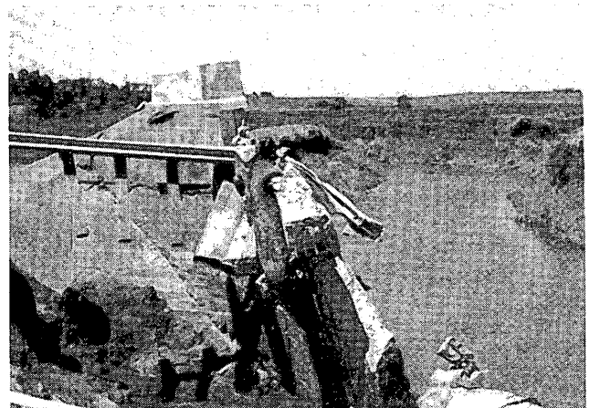
FIGURE 6 Site after flooding: (a) looking north along centerline of highway, (b) looking north (note scour hole upper right), (c) looking downstream (note blowout of channel), (d) south abutment (note piers failed and beams fell from abutment seat), and (e) looking upstream (note broad flat floodplain oversized for modern stream).
