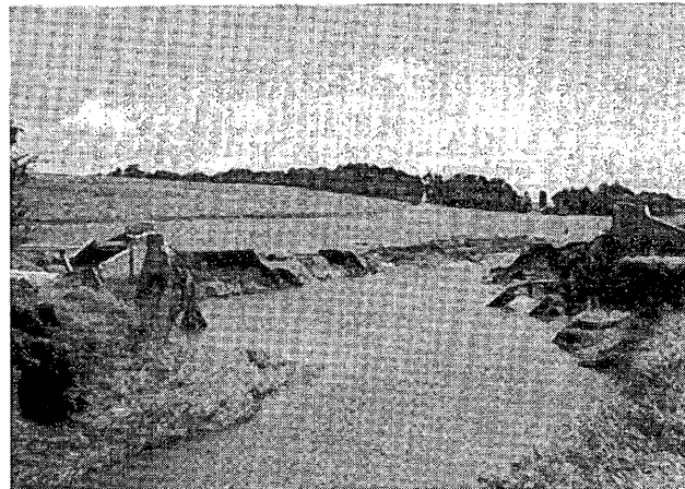
FIGURE 6 Site after flooding: (a) looking north along centerline of highway, (b) looking north (note scour hole upper right), (c) looking downstream (note blowout of channel), (d) south abutment (note piers failed and beams fell from abutment seat), and (e) looking upstream (note broad flat floodplain oversized for modern stream).
