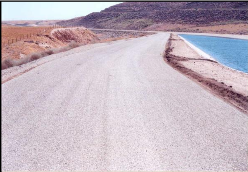
Slurry or Micro Surfacing – Low Volume Shoulders and Lots
