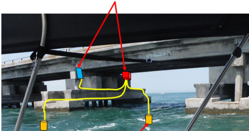
Transducers affixed to 66-inch dia. concrete cylinder piles a minimum of 2 feet below low tide level
