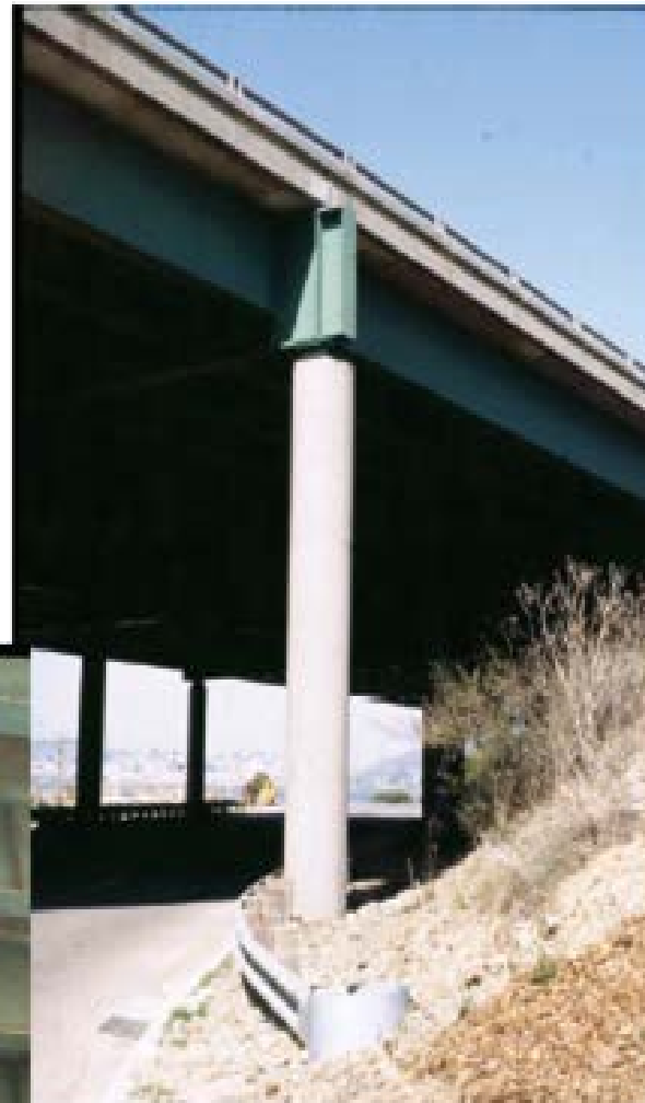
(b) Left: Replacement of existing steel bearing with lead-rubber isolator.
