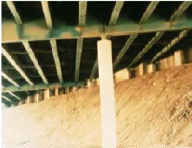
(a) Above: Single column with existing steel bearing before retrofit.
