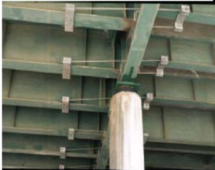
(a) Above: Single column with existing steel bearing before retrofit.
