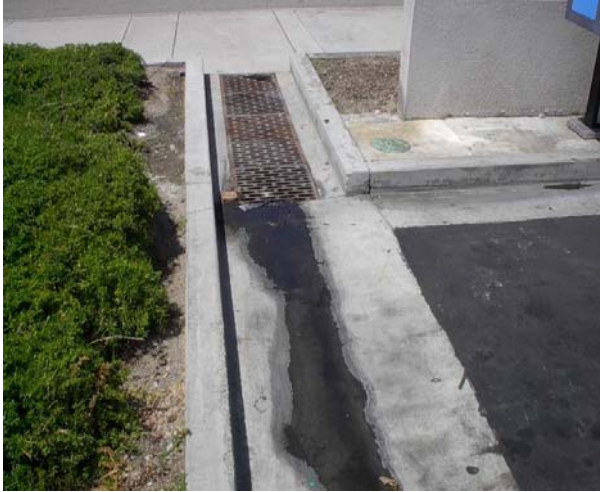
Figure 3: Wash Water from a Commercial Car Wash Discharging Down a Storm Drain–An Illicit Discharge.
