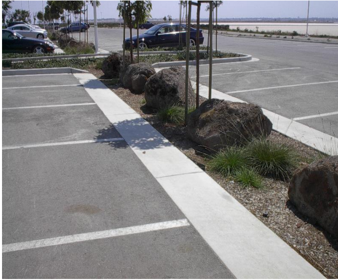
Figure 5: Infiltration Islands Help Reduce and Filter Pavement Runoff
